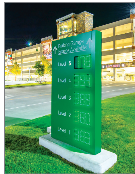
Walker Parking Consultants Wired and wireless sensors can monitor use of individual parking spaces throughout the facility to determine where open parking is available. That information is then wirelessly communicated and displayed via LED signage at key locations.
